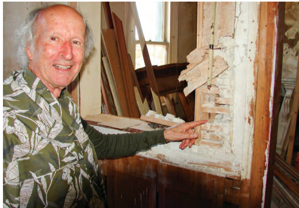
Architect Clive Cullen points to the old plaster system which will be replaced by more modern methods of construction.
